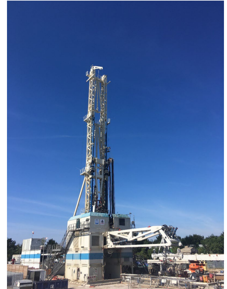
Figure 17: The drilling rig used for the United Downs Deep Geothermal Project (UDDGP)
